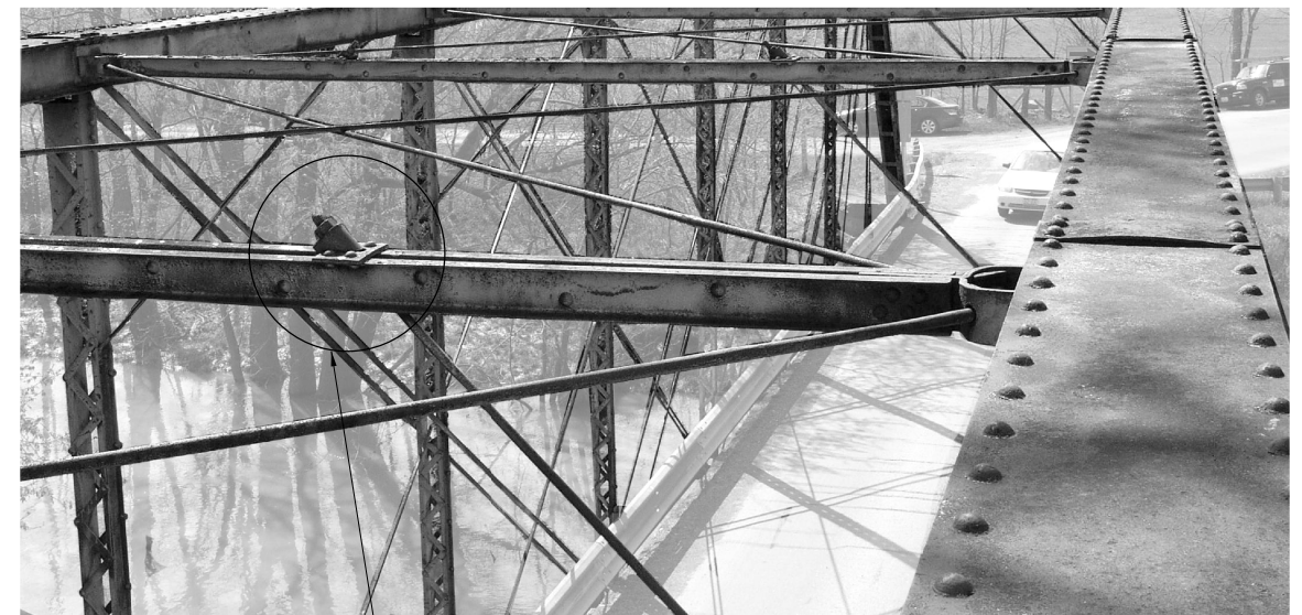
TYPICAL KNEE BRACE TO TOP STRUT CONNECTION **
