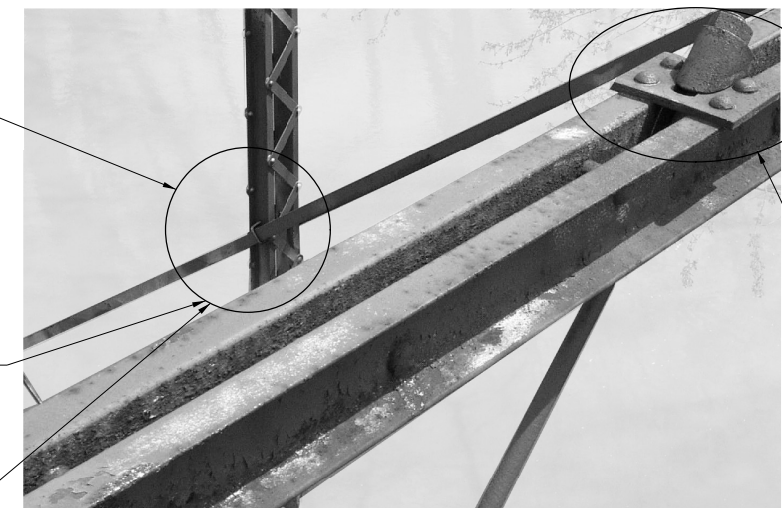
TYPICAL KNEE BRACE TO VERTICAL CONNECTION - SAVE AND REFURBISH CONNECTIONS. ** REPLACE RIVETS WITH HIGH STRENGTH BOLTS.
