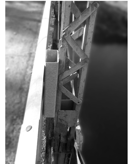
U5L5 - NORTH TRUSS, EAST SIDE
