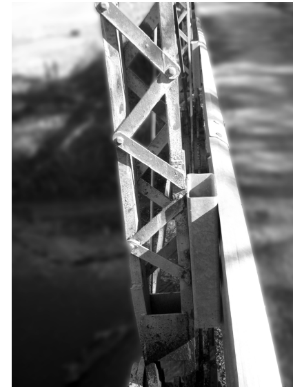
U5L5 - NORTH TRUSS, WEST SIDE
