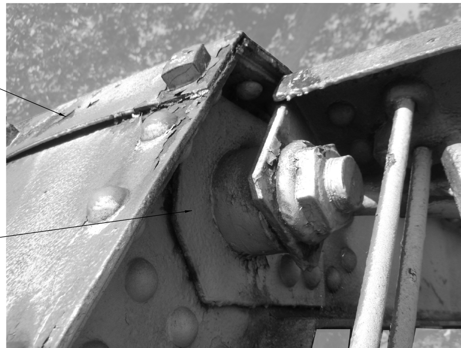
TYPICAL END POST TO TOP CHORD CONNECTION PIN 1.92" DIA. AT END. REPLACE ALL PINS AND NUTS WITH STAINLESS STEEL.
